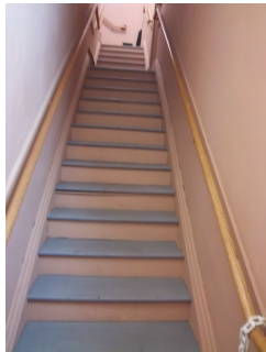
Back side stairway
