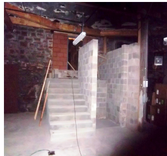
Stairs go alongside the lift.
