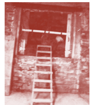
Interior coming from Temple Street
